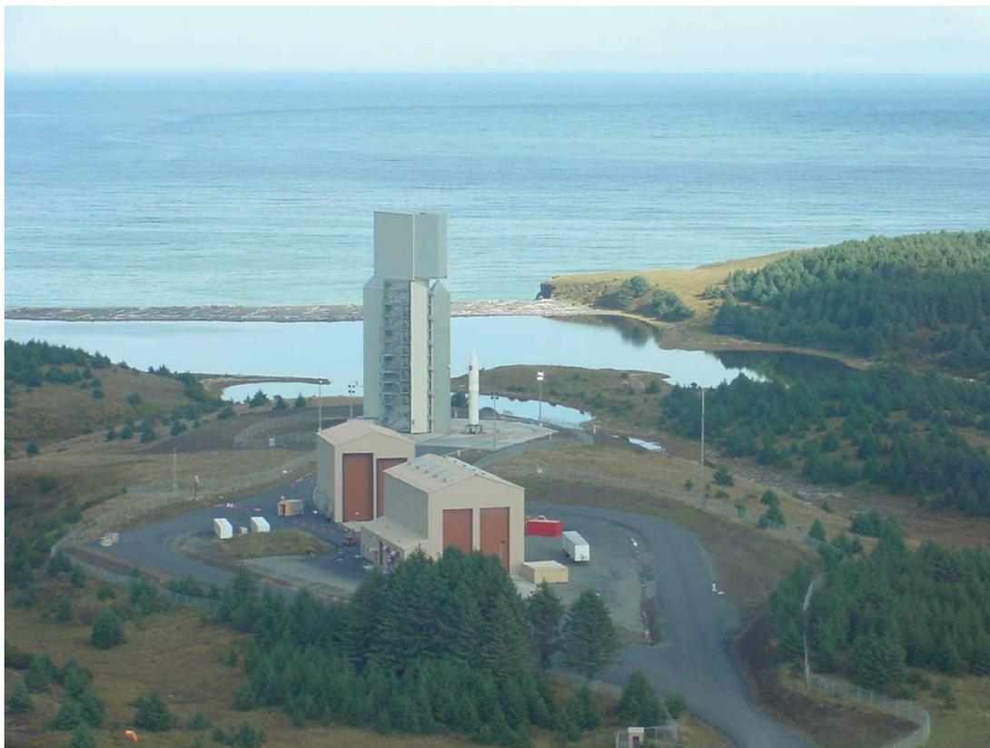
**Figure 3. Launch Pad Complex with from front to rear the IPF, SCAT, and LSS.**
