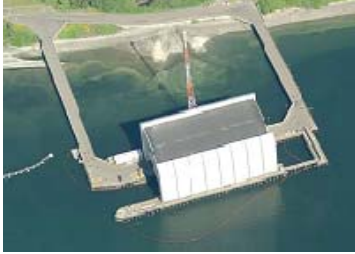
The existing EHW at Naval Base Kitsap Bangor
