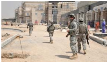
Army personnel near children's hospital construction project in Basra, Iraq, May 29, 2009. Concerned that the U.S. company Bechtel was mismanaging reconstruction funds in Iraq, government auditors in 2006 found that Bechtel was nearly $90 million over its original budget of $50 million and more than a year and a half behind schedule. U.S. Army photo by Sgt. Rodney Foliente
