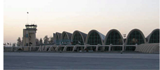
Figure 3. Kandahar International Airport served as the base of operations for the USGS airborne geophysical and remote sensing survey of Afghanistan. The terminal has seen significant renovations recently and will eventually be ready for civilian use.
